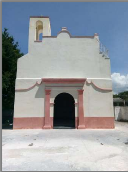
AREA: FACHADA PRINCIPAL
