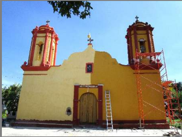
AREA: FACHADA PRINCIPAL
