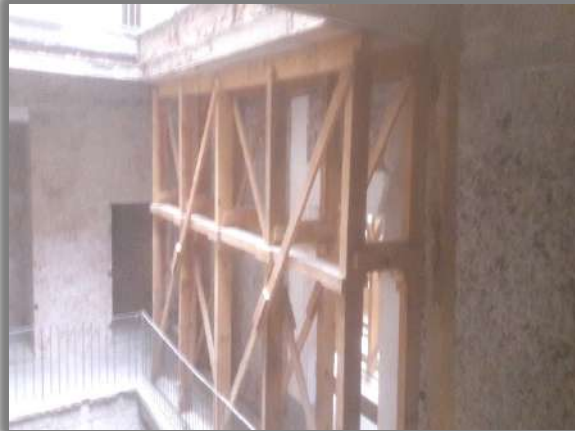
AREA: FACHADA INTERIOR
