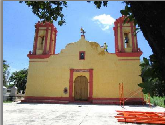
AREA: FACHADA PRINCIPAL
