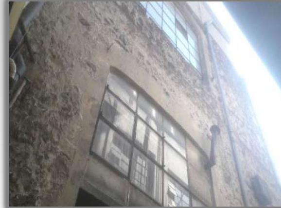
AREA: FACHADA INTERIOR
